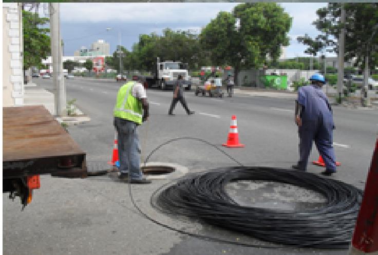
Kingston – Underground Fiber Optic Cable Installation
